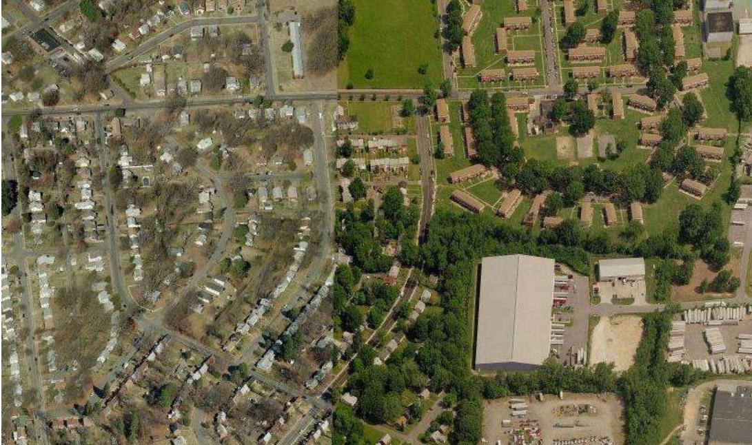
Figure 65. Insolation and aerial map of the Old Dominion Freight Warehouse.
