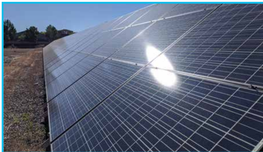
Mesa solar panel installation
