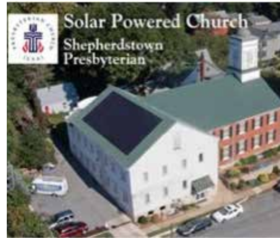
The Solar Holler model is the first of its kind and allows communities to go solar that otherwise would not have the financial resources. Its expanding access to solar, particularly in rural areas.
