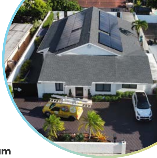
Co-op participant Richard Delgado's rooftop solar installation, provided by Goldin Solar.
