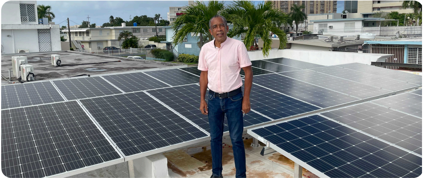
Puerto Rico solar homeowner Victor Santana on his roof next to his new system.
