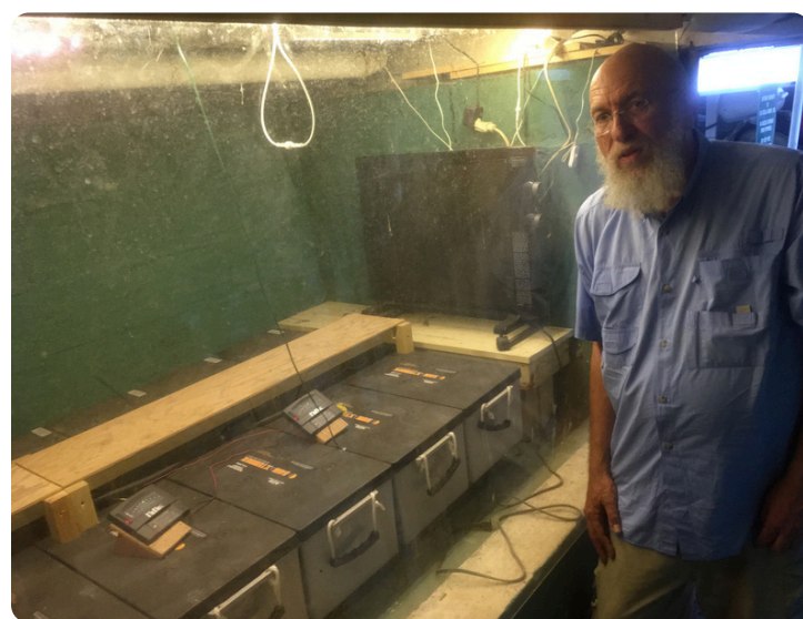
Virginia solar homeowner Scott Sklar with his Concorde Sun Xtender AGM bank.
